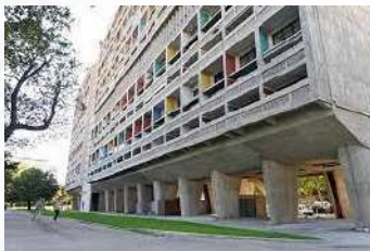
Unite d habitacion ( https://sitelecorbusier.com/en/unite-dhabitation/ )
