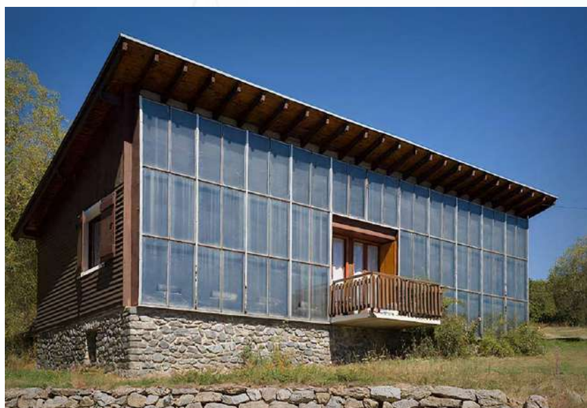
Jacques Michel's first Trombe Wall house in Odeillo. Image © Wikimedia Commons user OfHouses
